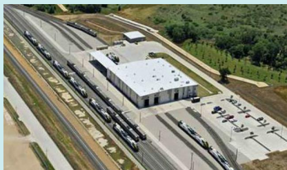
Photo: Denton County, TX Train Maintenance Facility
