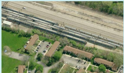
Photo: Metra Electric District - Richton Layover
