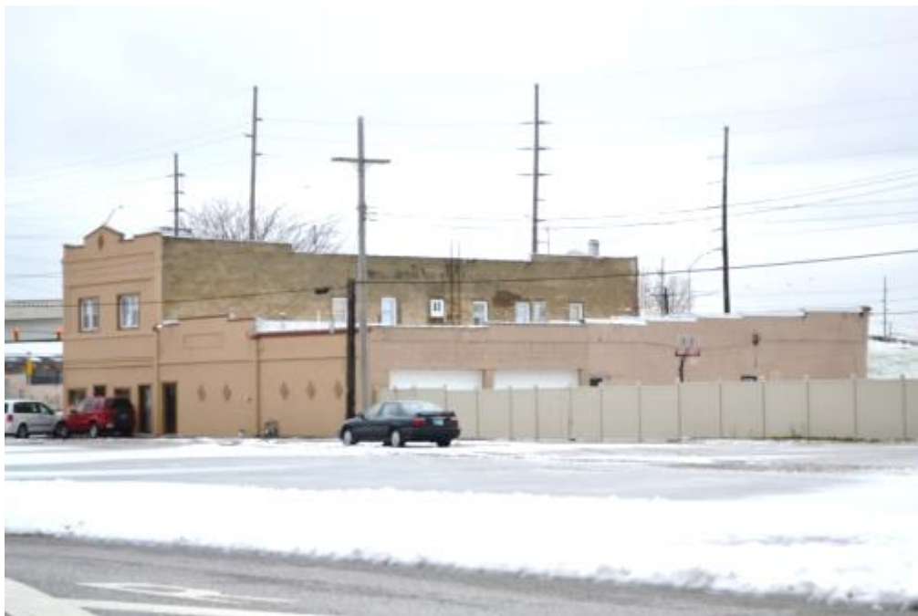
Figure 5-39: Stucco Sheathing on southwest sides of 424 and 422 Willow Court (view northwest)
