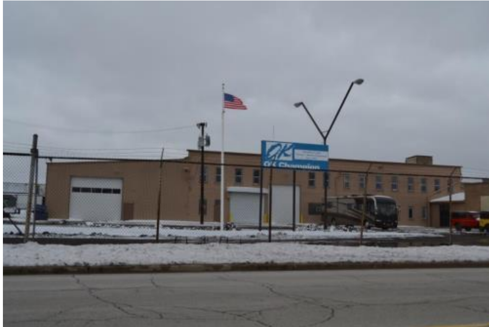
Figure 5-54: Two-story Section of the O.K. Champion Building (view southeast)
