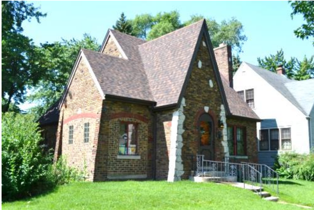
Figure 5-4: 266-268 Oakwood Street (view southeast)
