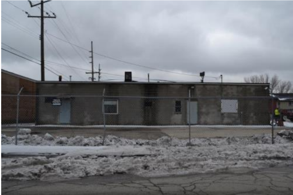
Figure 5-48: Concrete Block Aldobilt Building (view south)
