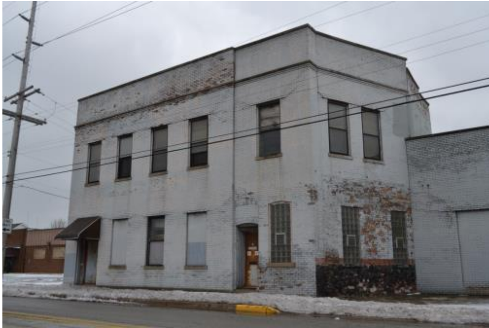
Figure 5-66: 304 Gostlin Street (view southeast)
