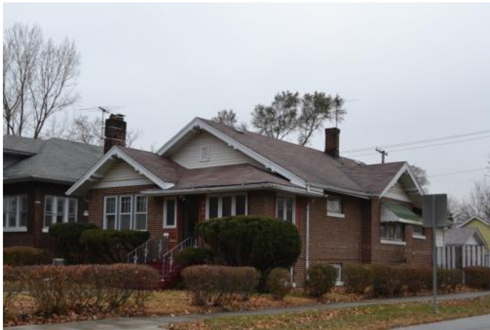
Figure 5-11: 267 Dyer Boulevard (view northwest)
