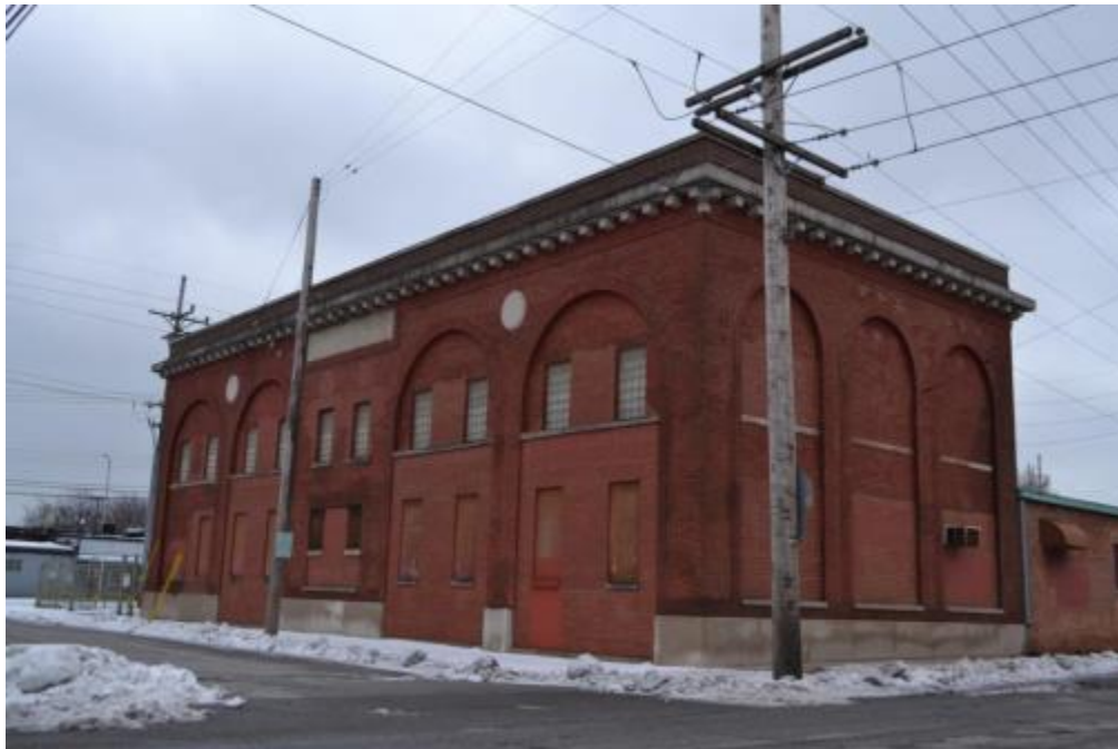
Figure 5-64: NIPSCO Substation (view southeast)
