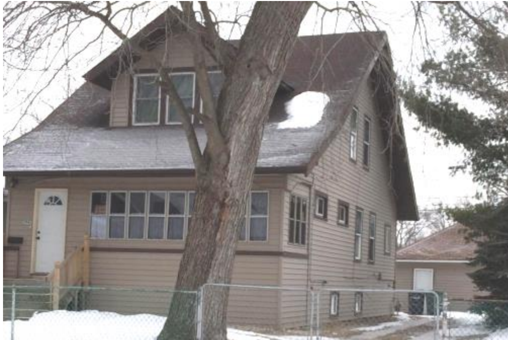
Figure 5-21: 5945 Park Place (view northeast)
