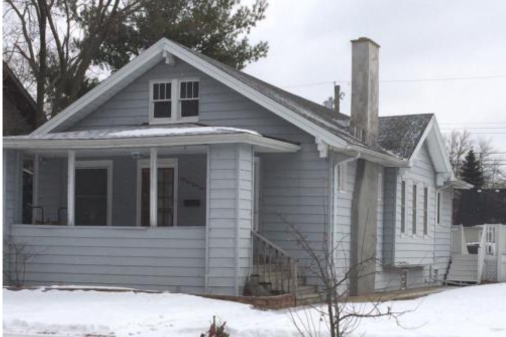
Figure 5-20: 5949 Park Place (view northeast)
