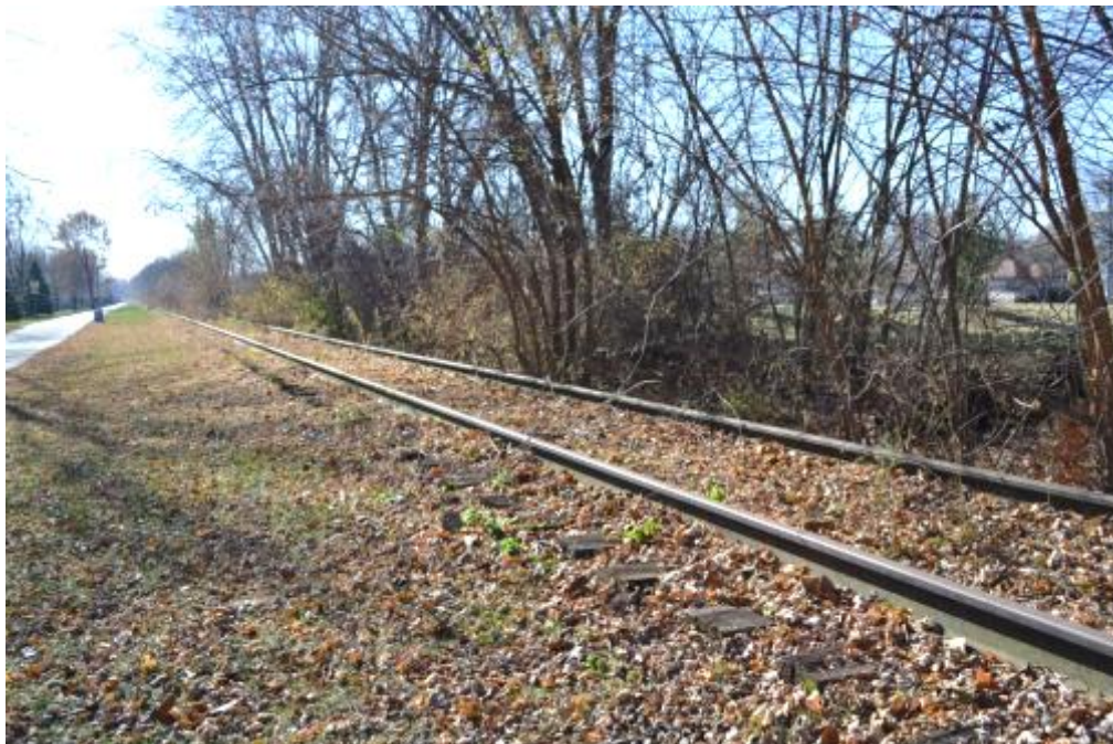
Figure 5-2: Monon Railroad Segment in Munster (view south)
