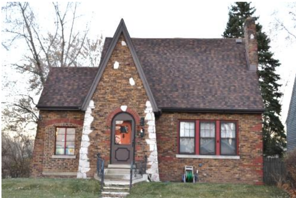
Figure 5-5: 266-268 Oakwood Street (view south)
