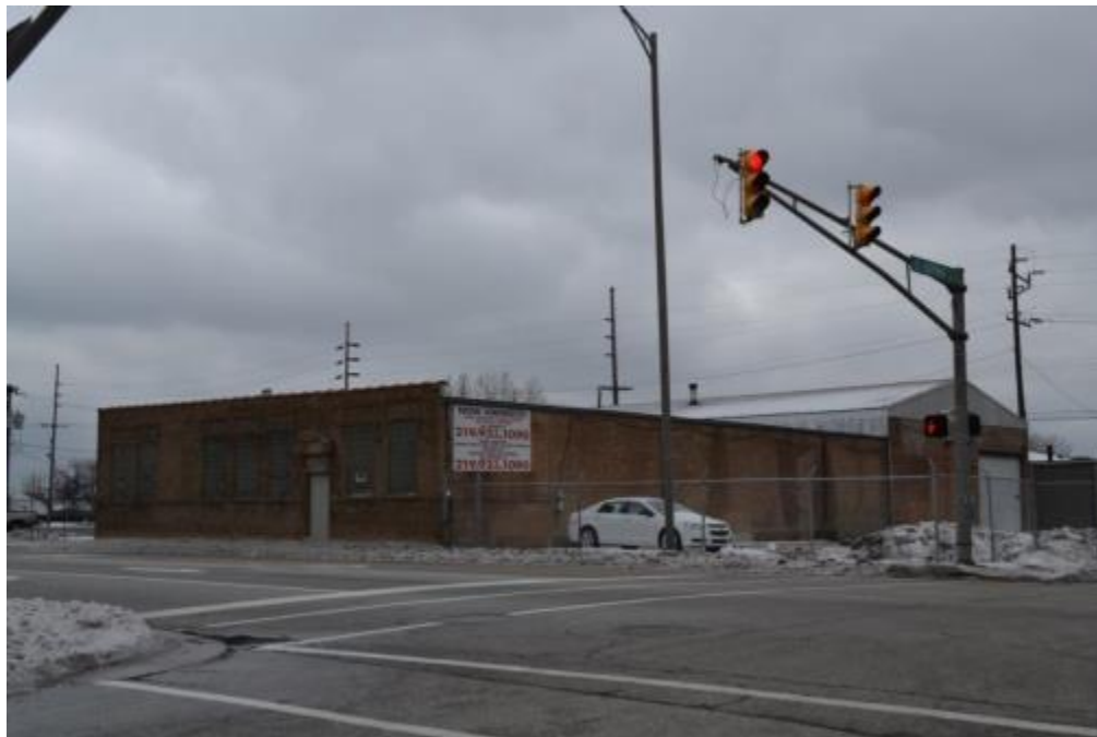
Figure 5-47: “L” Shaped, One-story, Brick Aldobilt Building (view southwest)
