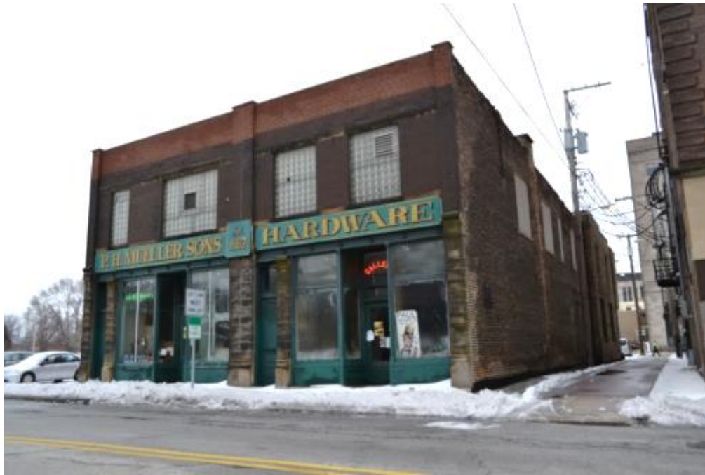
Figure 5-36: 416-418 Sibley Street (view south)
