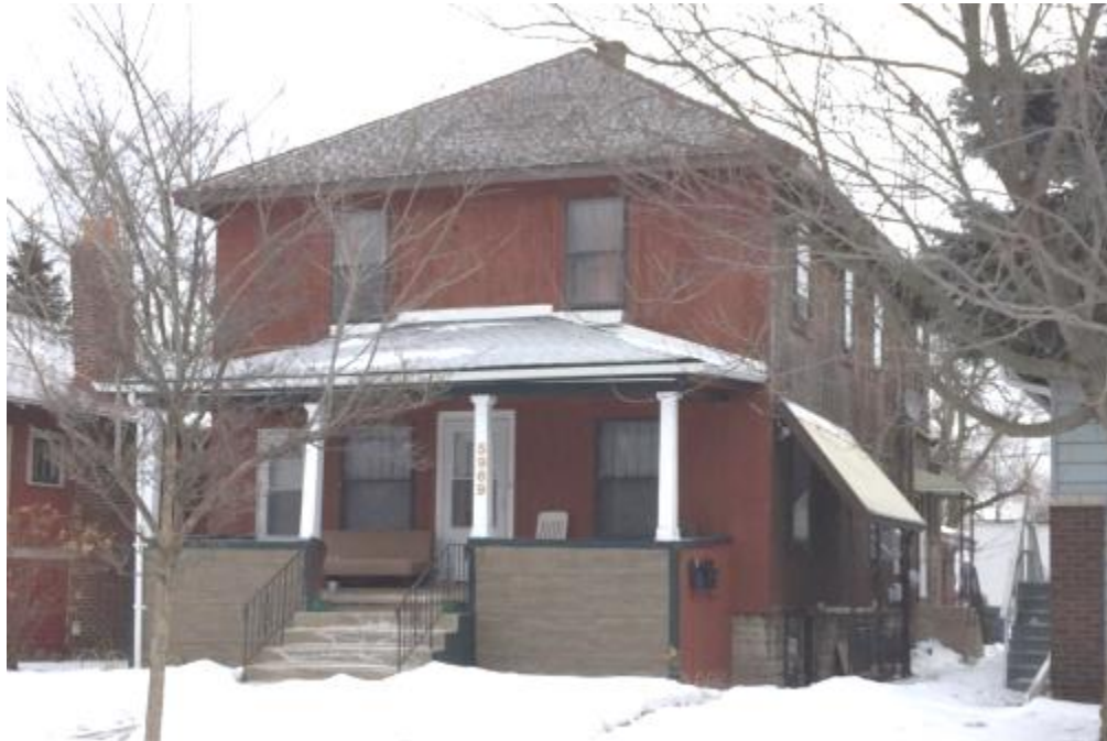
Figure 5-15: 5969 Park Place (view northeast)
