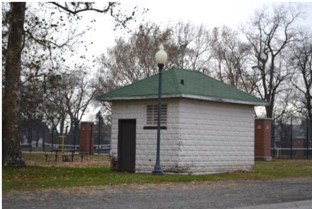
Figure 5-25: Harrison Park Utility Shed (view northwest from Lyman Avenue)
