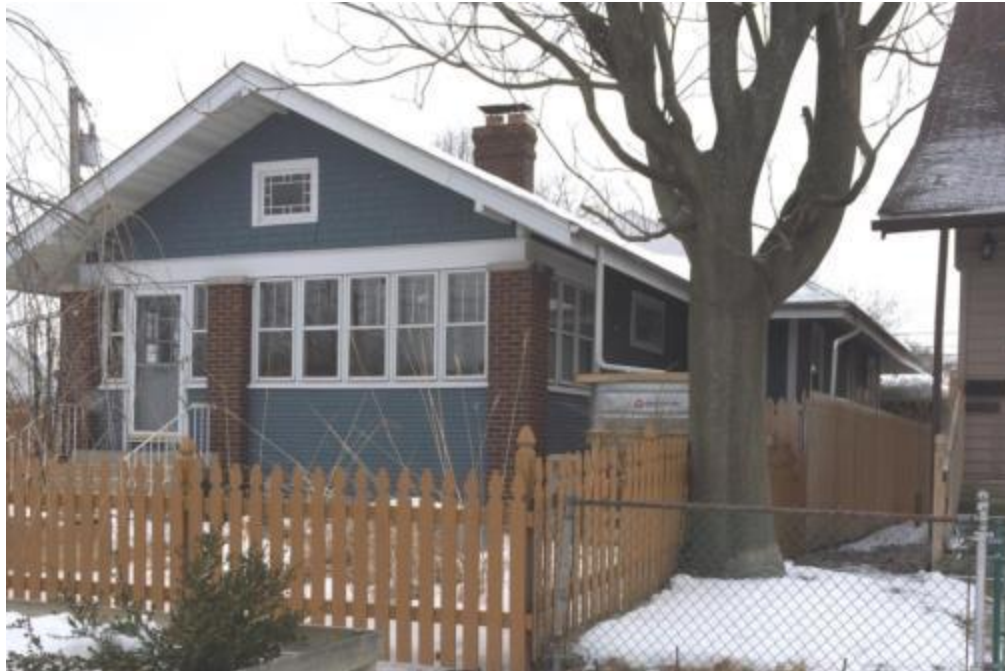
Figure 5-22: 5943 Park Place (view northeast)
