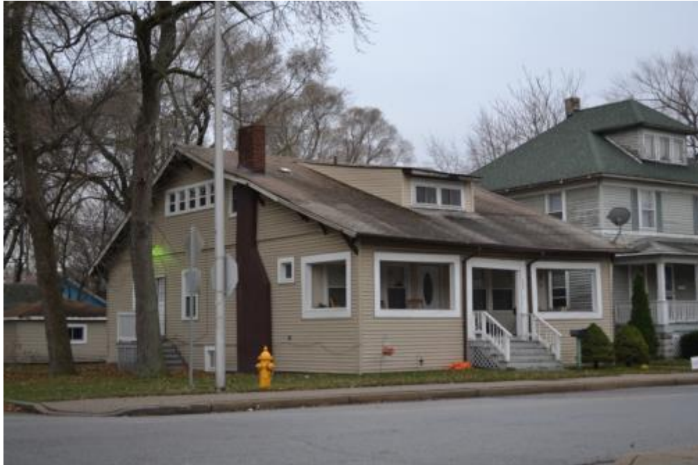
Figure 5-13: 266 Highland Street (view southwest)
