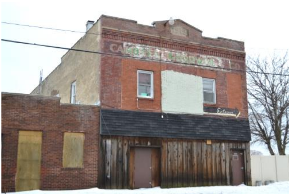
Figure 5-40: Northeast Side of 422 Willow Court (view west)
