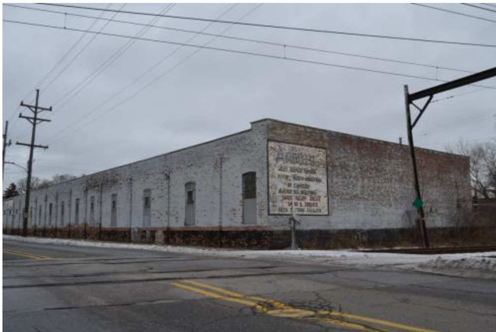
Figure 5-67: 304 Gostlin Street (view northeast)
