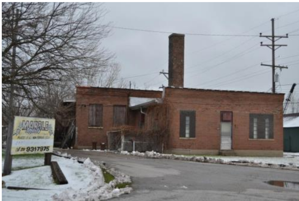
Figure 5-62: One-story Building at Standard Indiana Bulk Oil Yard (view northeast)
