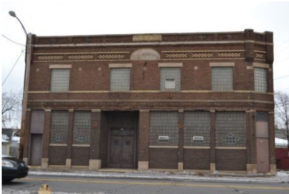
Figure 5-68: Polish Army Veterans' Post (view north)
