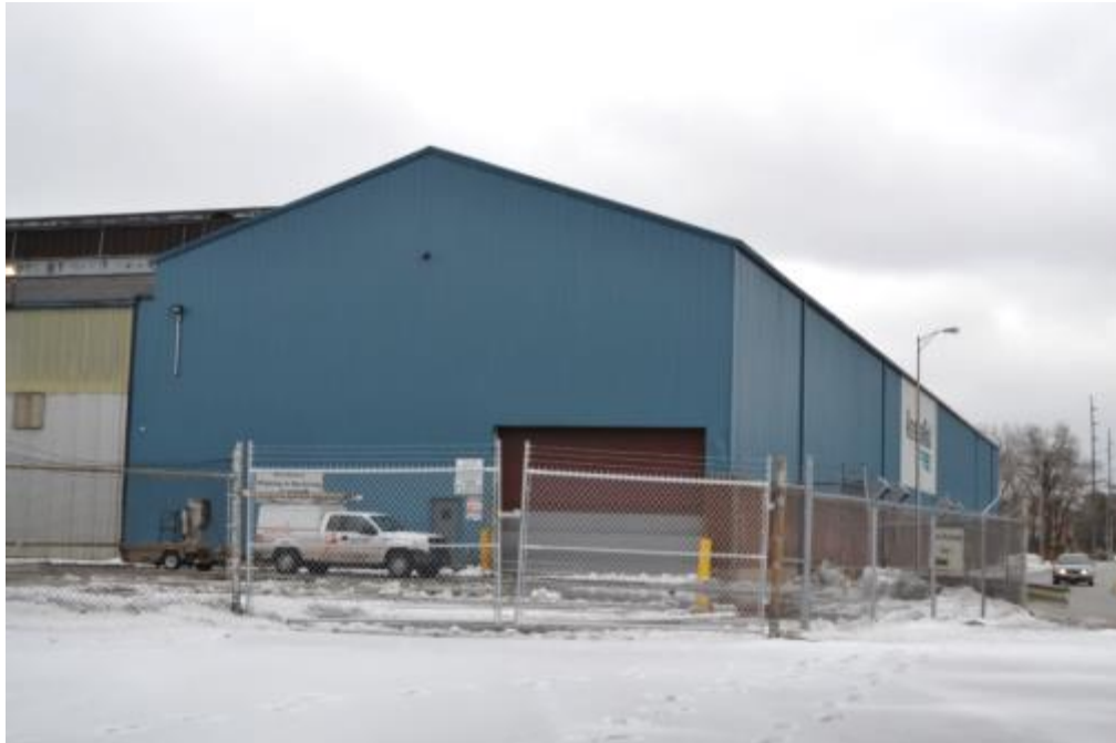
Figure 5-44: Building Constructed in 1960s (view south)
