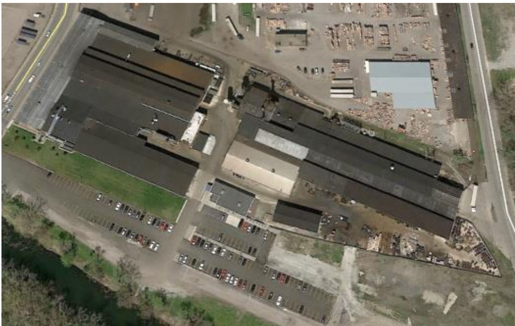
Figure 5-43: Google Earth Image of 4831 Hohman Avenue Depicting its Current Condition
