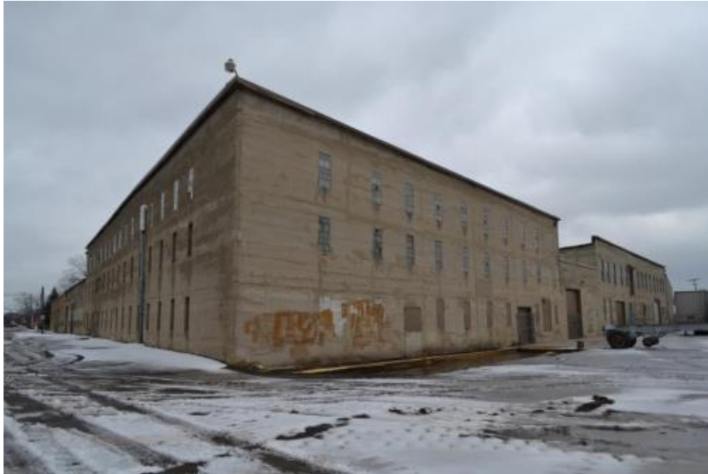
Figure 5-53: Three-story Section of the O.K. Champion Building (view southeast)
