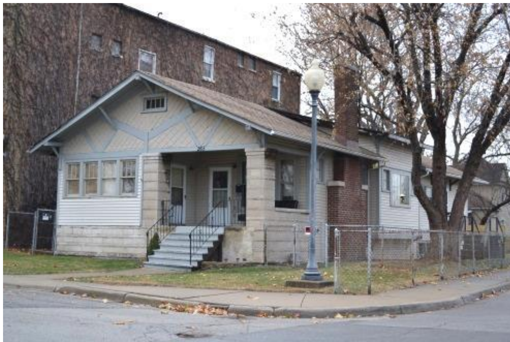
Figure 5-27: 265 Webb Street (view southwest)
