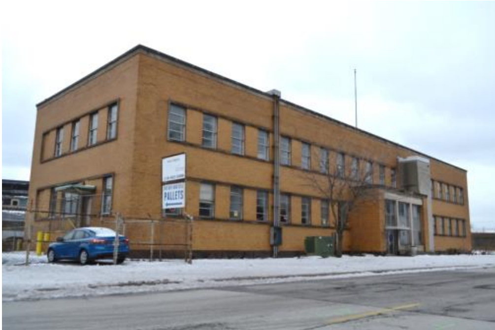
Figure 5-50: Office Building at 420 Hoffman Street (view southwest)
