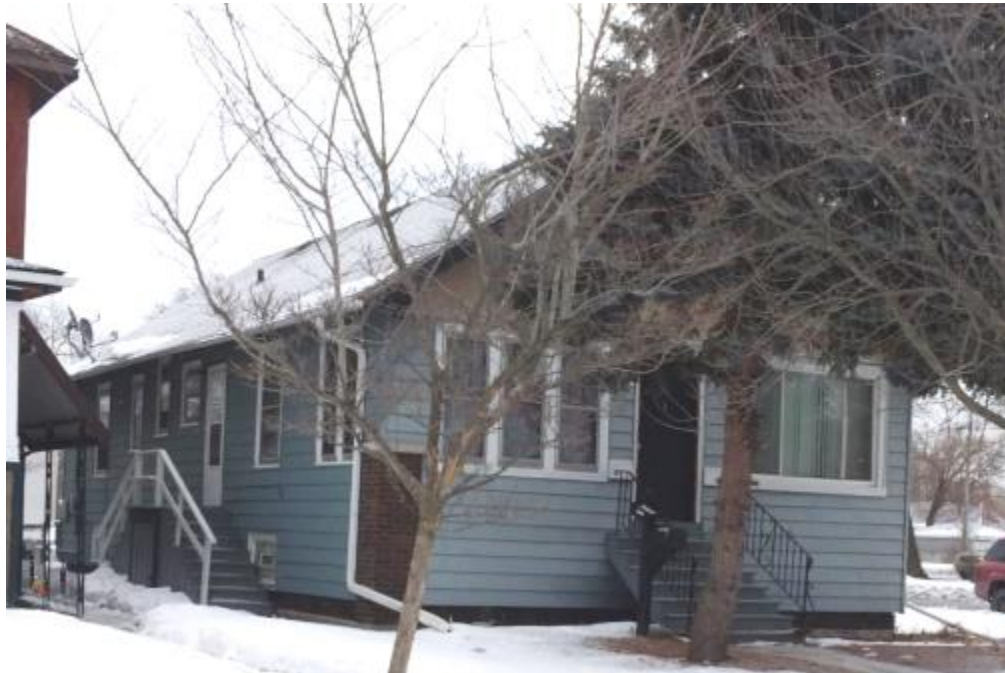
Figure 5-14: 5973 Park Place (view southeast)
