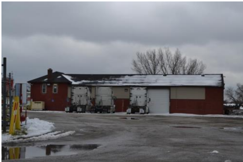
Figure 5-49: Office/Warehouse Building (view southwest)
