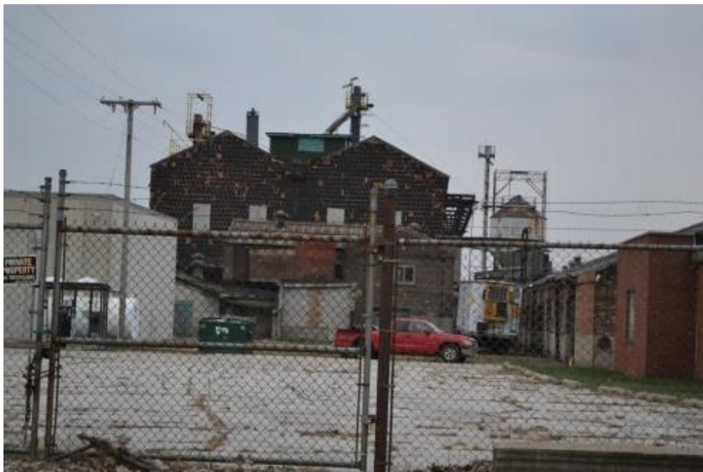
Figure 5-59: Federal Cement Tile Company Sand Storage Building and Coal Room (view south)
