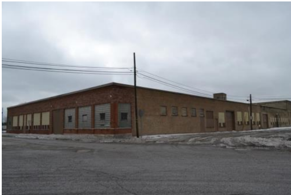
Figure 5-52: One-story Section of the O.K. Champion Building (view southwest)
