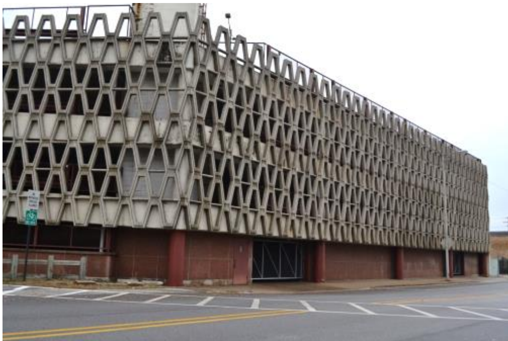
Figure 5-35: Minas Parking Garage, West and South Sides (view southeast)
