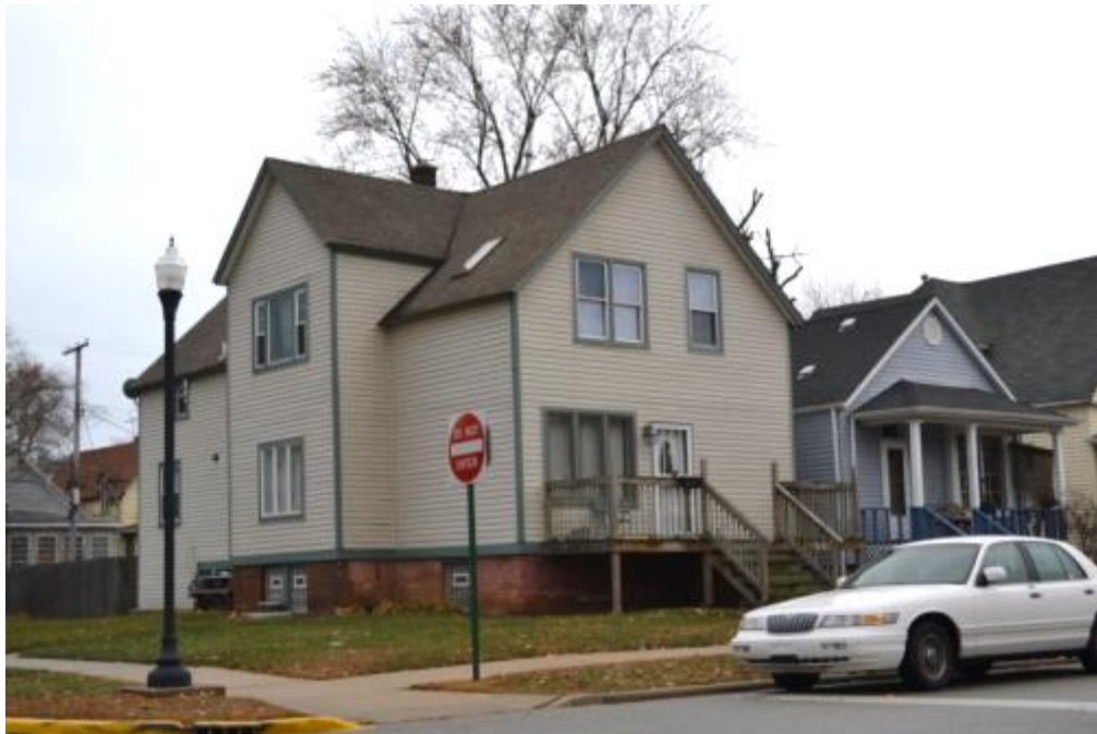
Figure 5-29: 256 Williams Street (view southwest)
