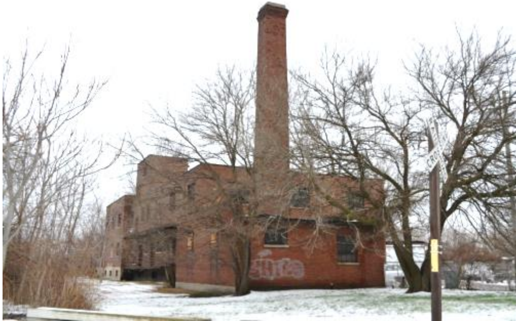
Figure 5-63: Two-story Building at Standard Indiana Bulk Oil Yard (view northwest)
