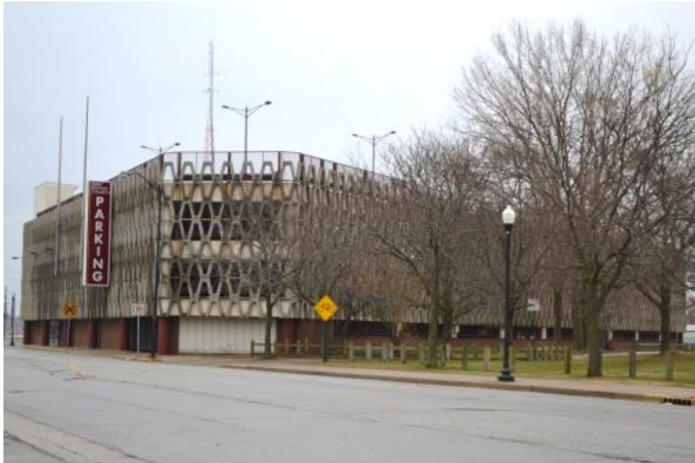
Figure 5-34: Minas Parking Garage, North and West Sides (view southeast)
