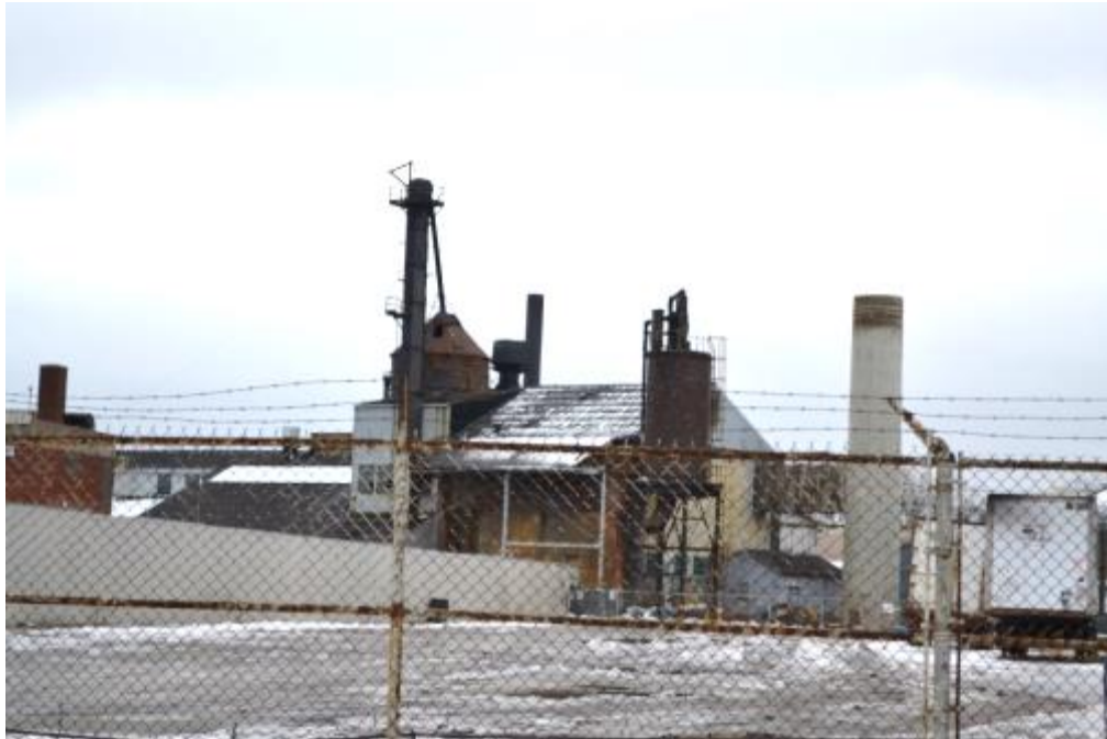
Figure 5-46: Other Buildings and Smoke Stack at the Simplex Facility (view southwest)
