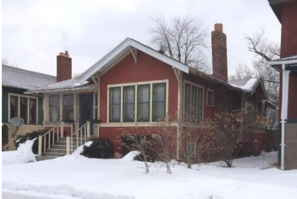
Figure 5-16: 5967 Park Place (view northeast)
