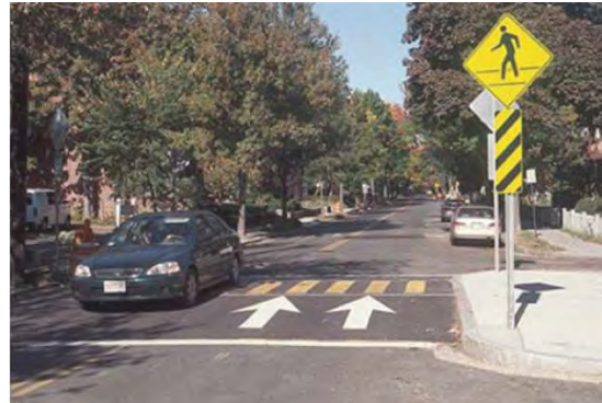
Speed table doubling as a raised crosswalk
