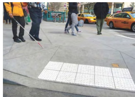
Crossing ramp with a truncated dome surface
